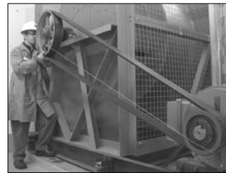
Using a string to check alignment
