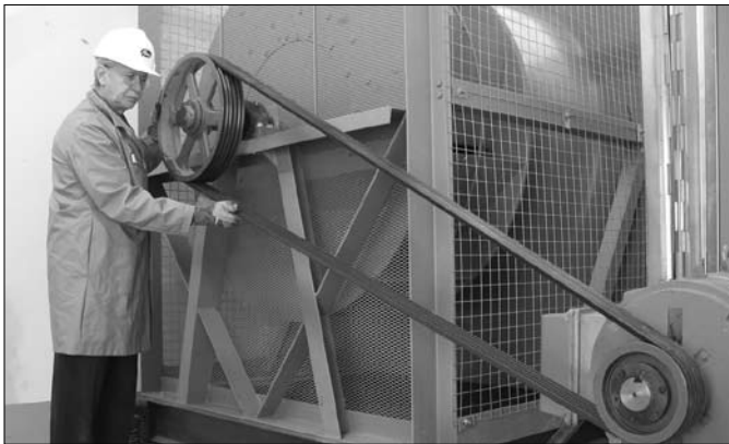
Begin by inspecting the belt
