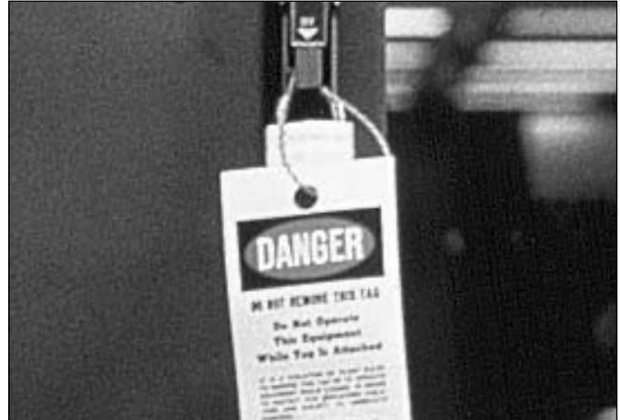
Turn off power, lock controls and tag
