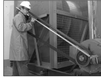
Using a straight edge to check alignment
